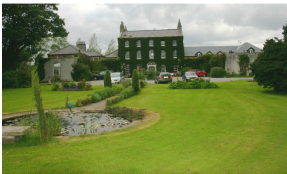
Fig.C-30: Belcamp Hutchinson (picture curtesy of NIAH)
