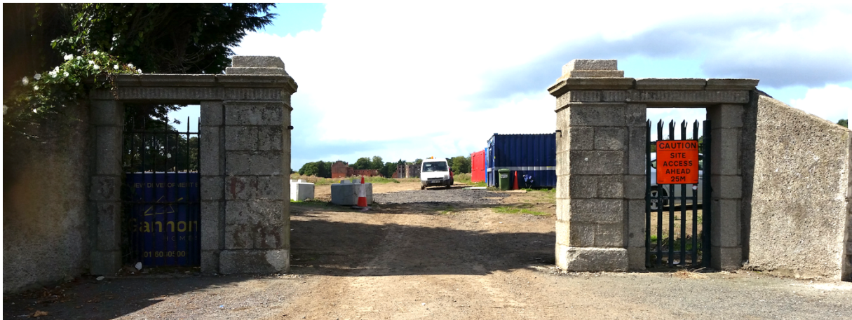
Fig.C-29: Balgriffin Entrance Gates – currently in storage
