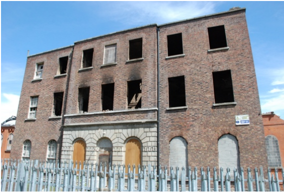
Fig.C-03: Belcamp Hall, west (front) elevation
