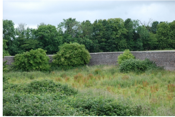
Fig.C-17: north wall, internal view of east bend
