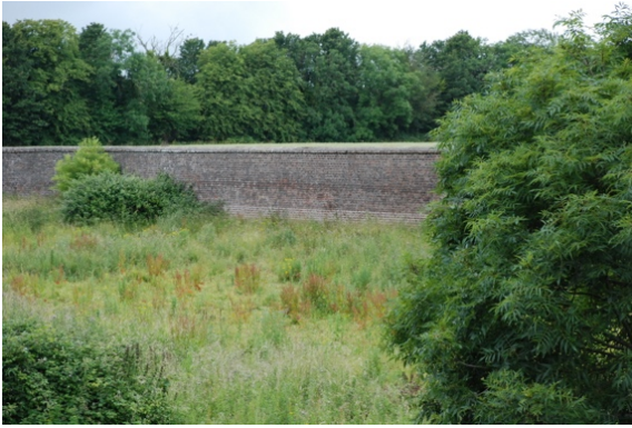
Fig.C-16: north wall, internal view looking west
