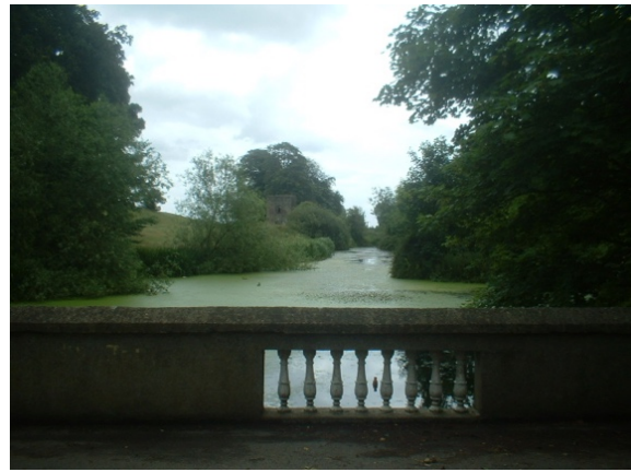
Fig.C-28: Bridge (Causeway), looking east
