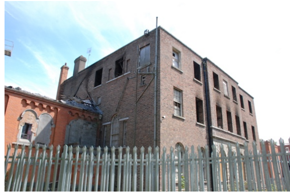
Fig.C-04: Belcamp Hall, north (side) elevation
