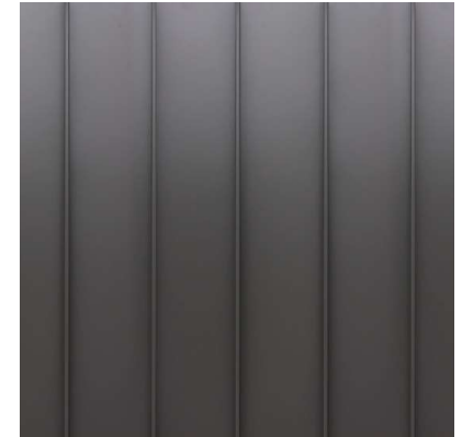
Fig . 38 – Example of standing metal seam claddings
