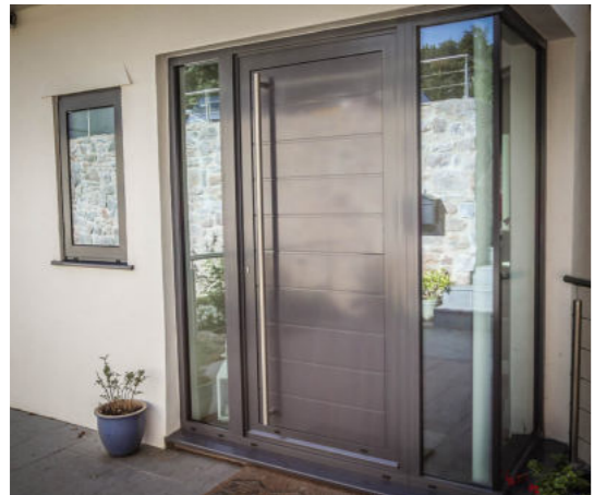
Timber entrance door
