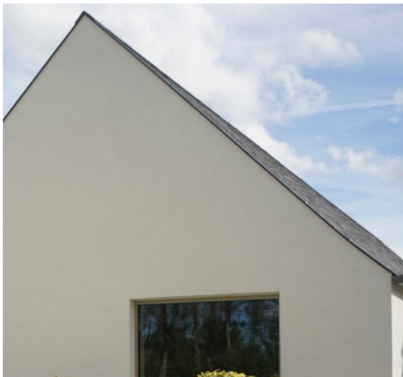
Flush eaves detail to roofs
