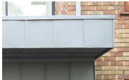
Standing seam metal entrance canopy
