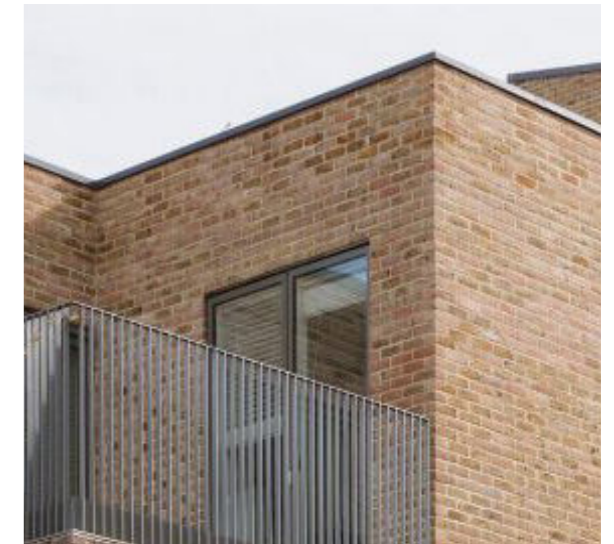
Dark metal windows and coping detail
