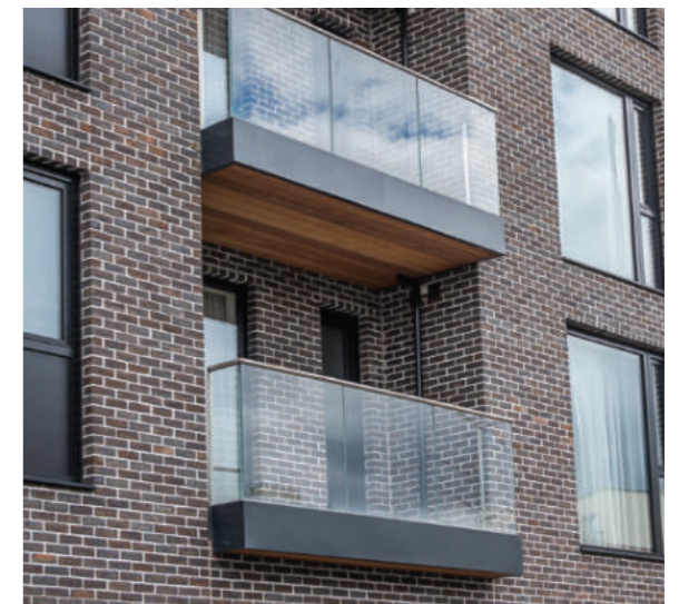
Glass balustrade to balconies
