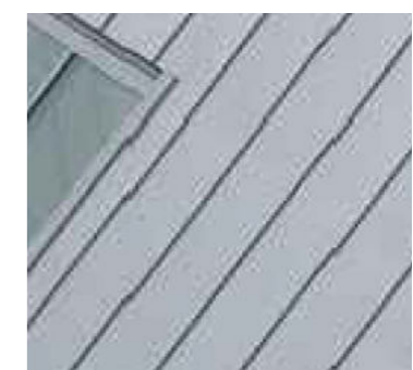
Metal cladding to stairs
