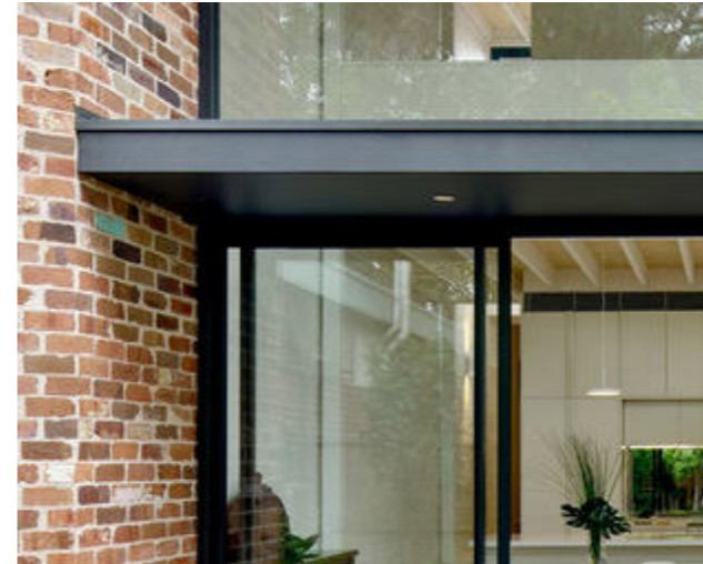
Metal entrance canopy
