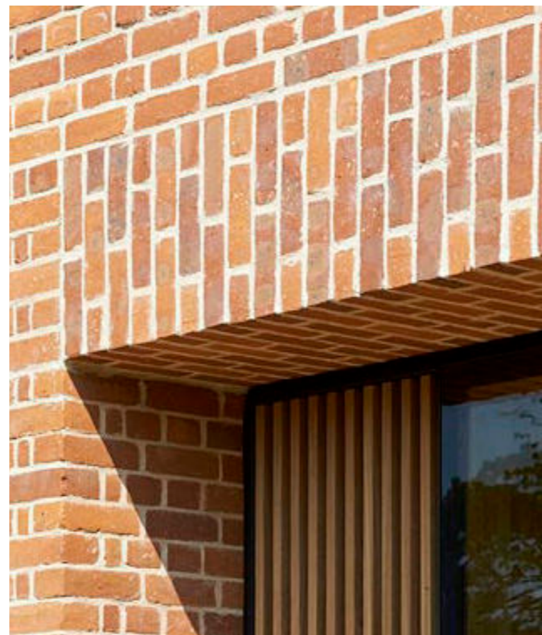
Examples of brick articulation detailing and high quality finishing.
