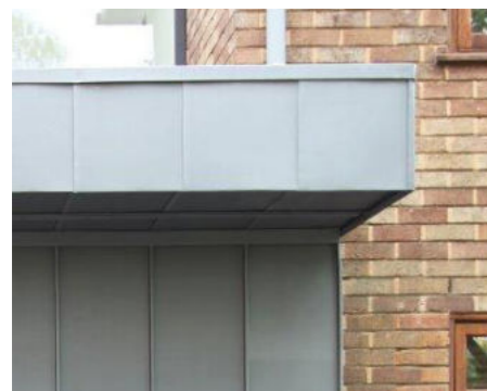
Metal entrance canopy
