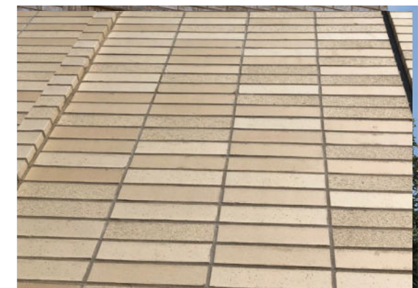
Stackbond brick detail to facade
