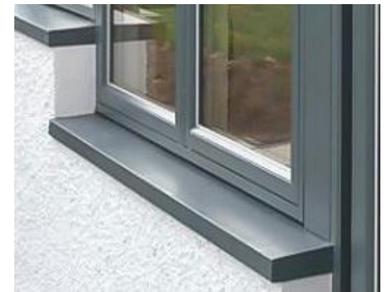
Pressed metal cill and window
