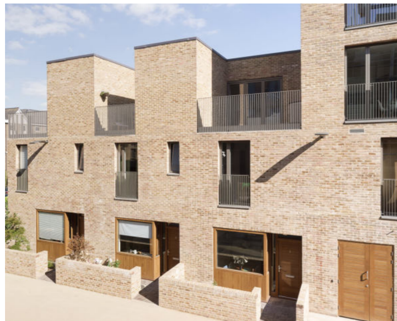
Recessed balconies with metal guarding Light ochre brick colour
