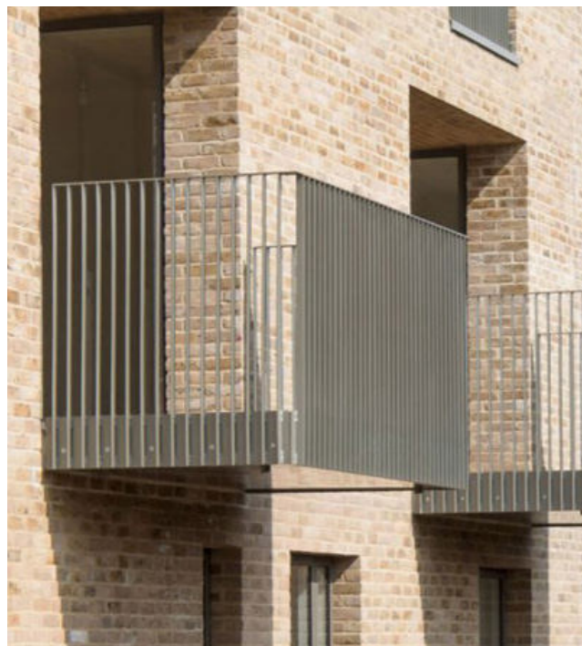
Example of metal guarded semi-recessed balconies
