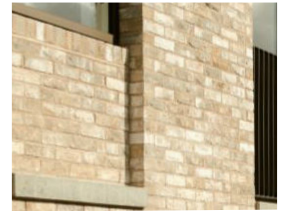
recessed brick panel detail
