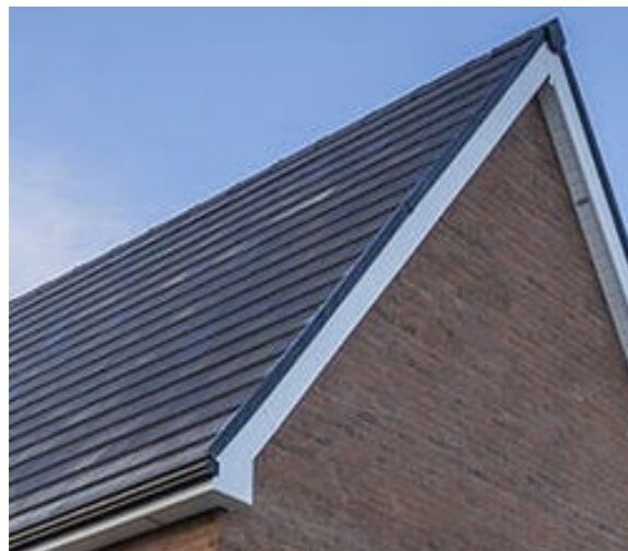
Dark concrete tile to roofs
