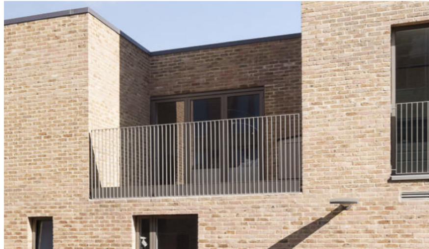
Powdercoated aluminium windows and metal guarding detail
