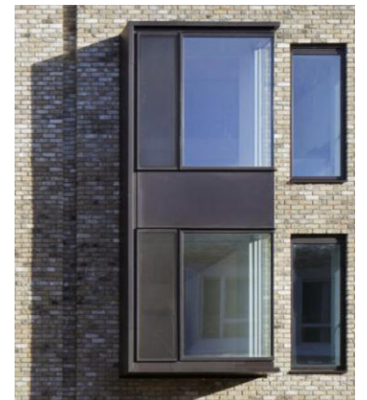
Dark metal bay window to gables
