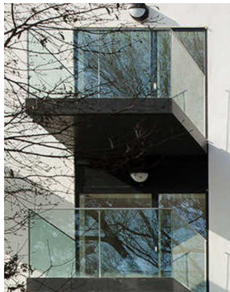
Glass guarding to balconies
