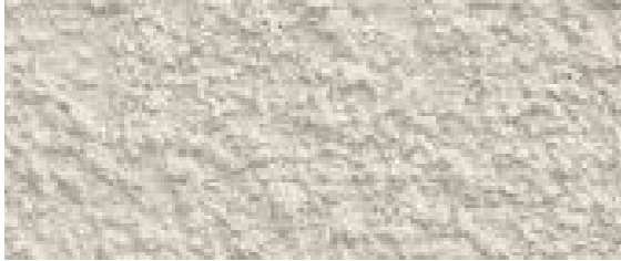
Rendered finish to panels on facade
