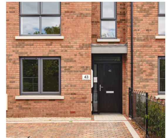
Painted entrance doors to own door units
