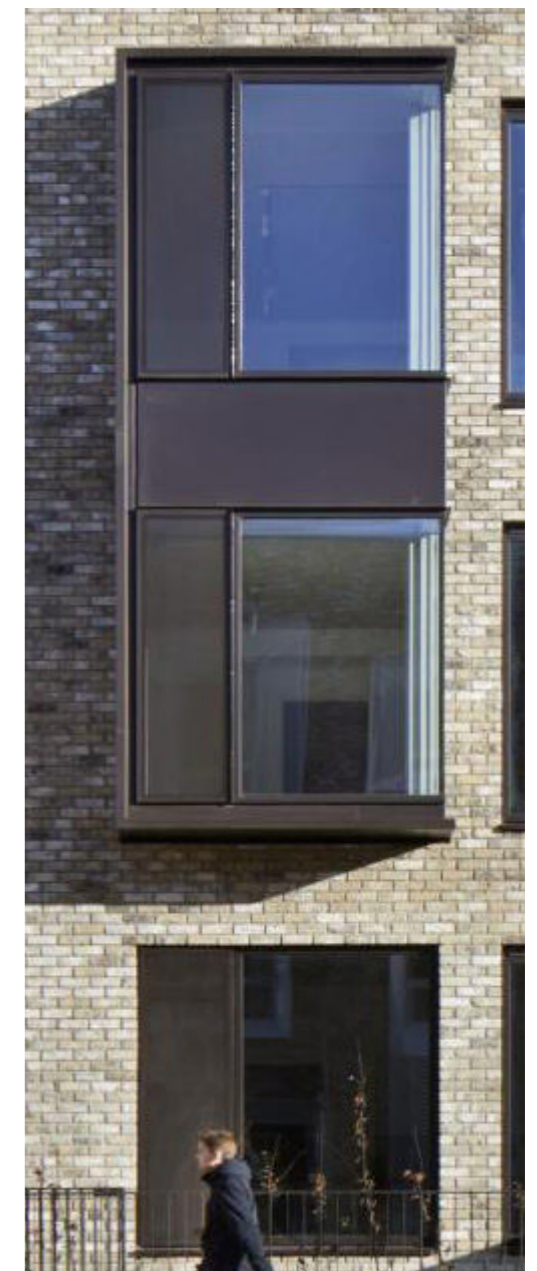
Metal bay window and brick detail.
