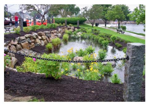
Figure 9.7 Typical Bioretention Garden
