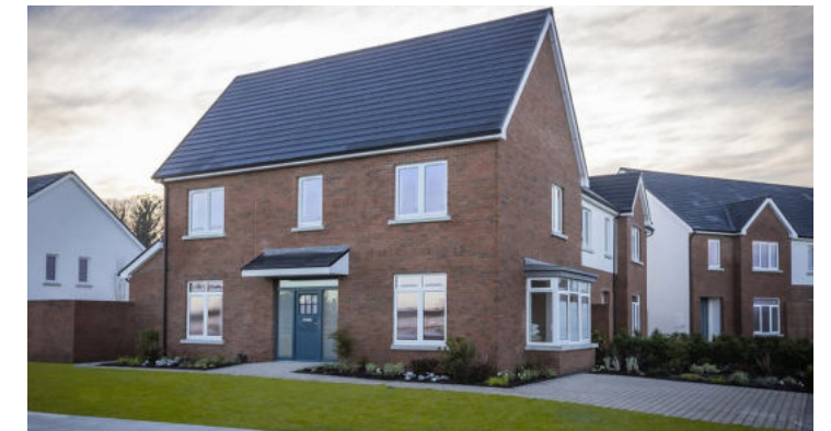
PHASE 1 HOUSING IN BELCAMP
