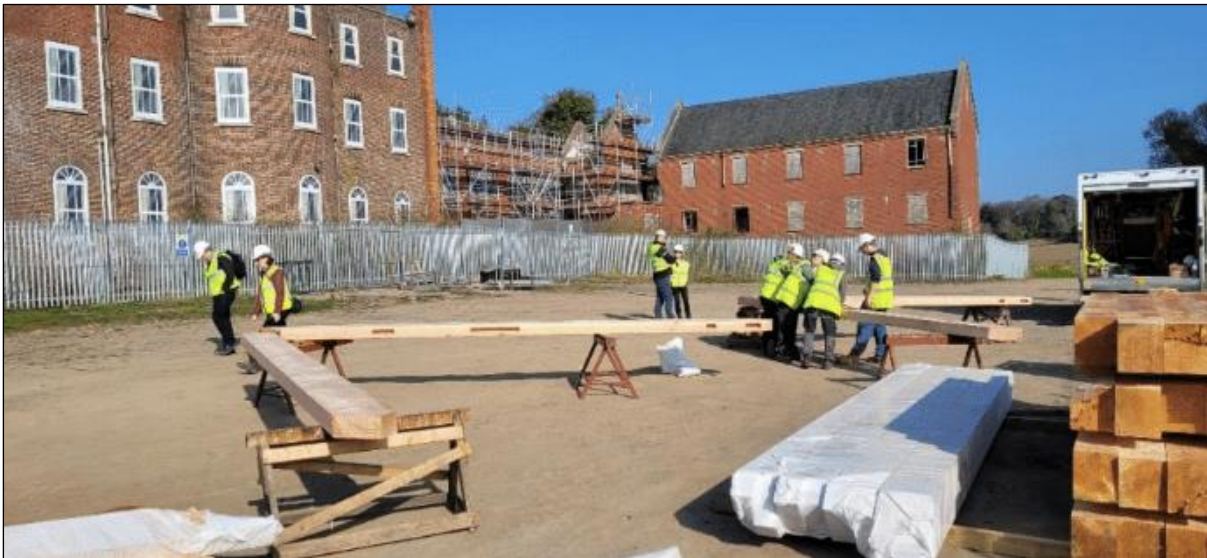
Figure 4: Chapel roof repairs underway
